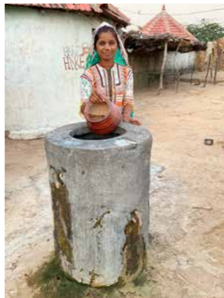
Figure -284 Traditional water tank
